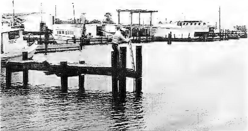
Figure 10. Staff being replaced at Fulton Harbor public boat ramp, Aransas Bay (see Staff 5, Chart G, Appendix B)
